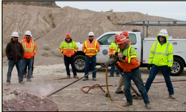
Using sink and jack leg drills
